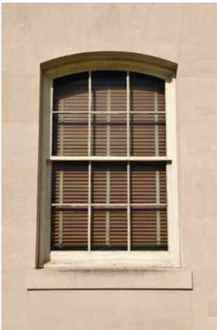
Typical Wood Framed Double-Hung Window
