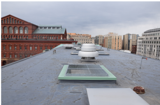
Slow Slope Roof Covering - Single-Ply PVC
