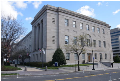
Building B Southwest view
