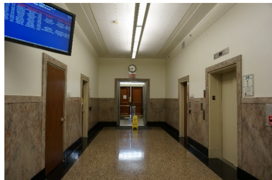
Historic Marble Slabs at Main Corridor
