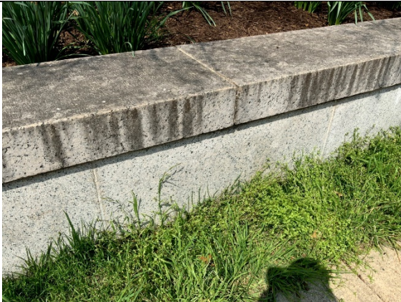
Figure S- 20 Site Retaining Wall
