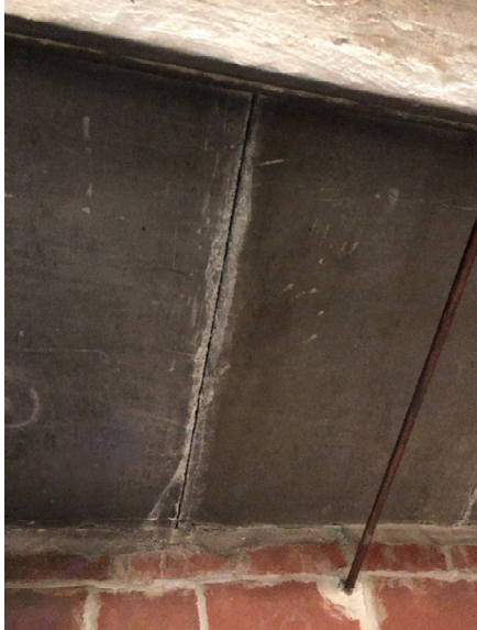
Figure S-8 Underside of Roof Precast Plank
