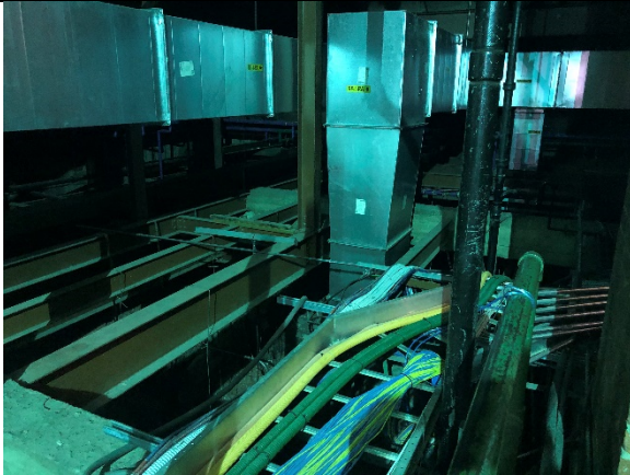
Figure S-6 Exposed Steel Framing and Ceiling in Attic
