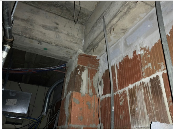
Figure S-5 View of Steel Column Wrap and Beam Encasement
