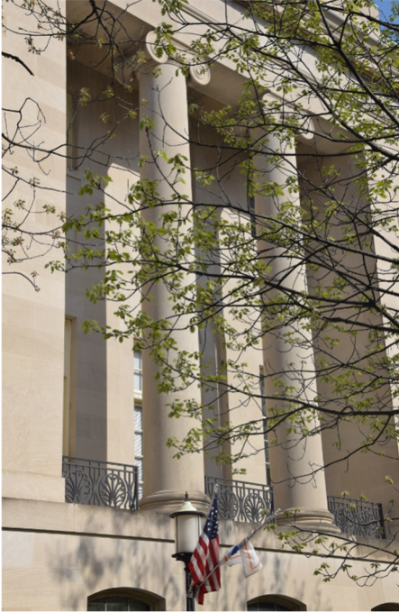
West Elevation Balconies
