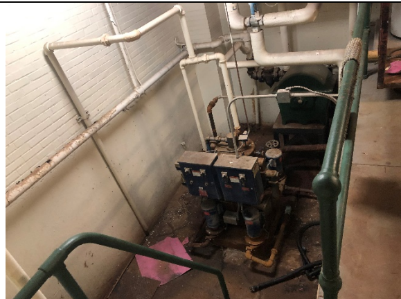
Figure S-10 View of Equipment Pit in Basement SOG
