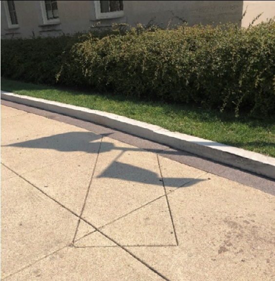
Figure S- 3 Sidewalk Joints Above Basement Grade Beams
