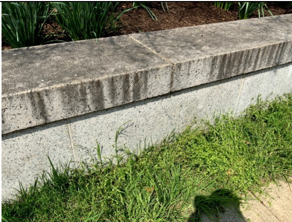
Figure S- 20 Site Retaining Wall (RETW-B01SNE-001) (CGCG-B01SNE-001, CGCG-B01SSE-001, CUGU-B01000-001)
