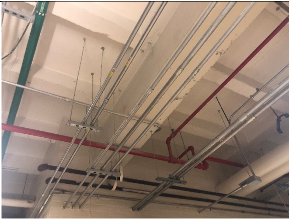
Figure S-4 View of Underside of slab from Basement
