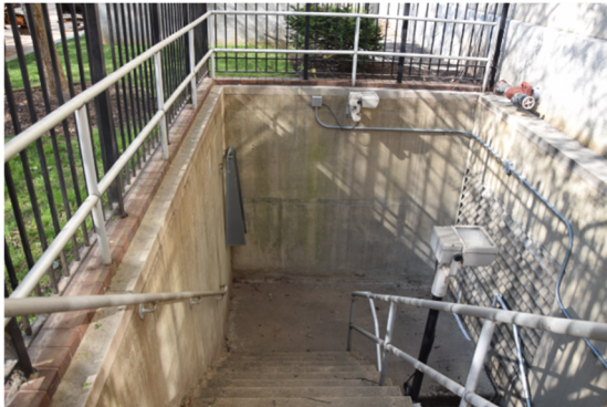
Basement Service Entrance at West Grounds
