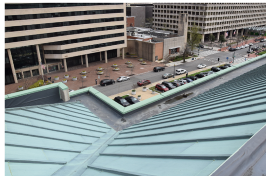
Copper Standing Seam Roof System
