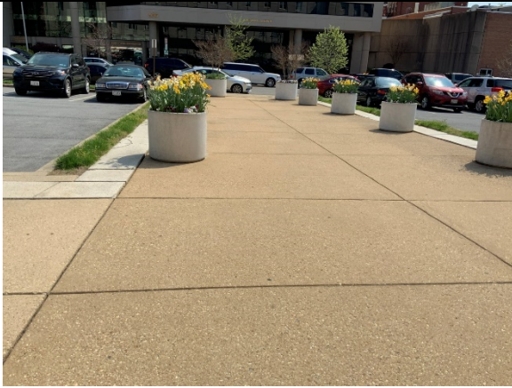
Figure S- 18 Sidewalk Paving On East Side
