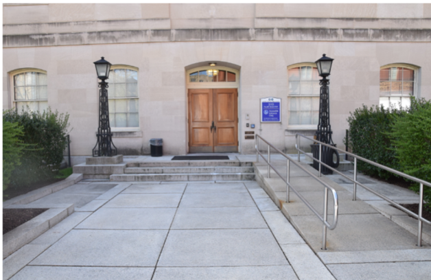
North Elevation Accessible Ramp
